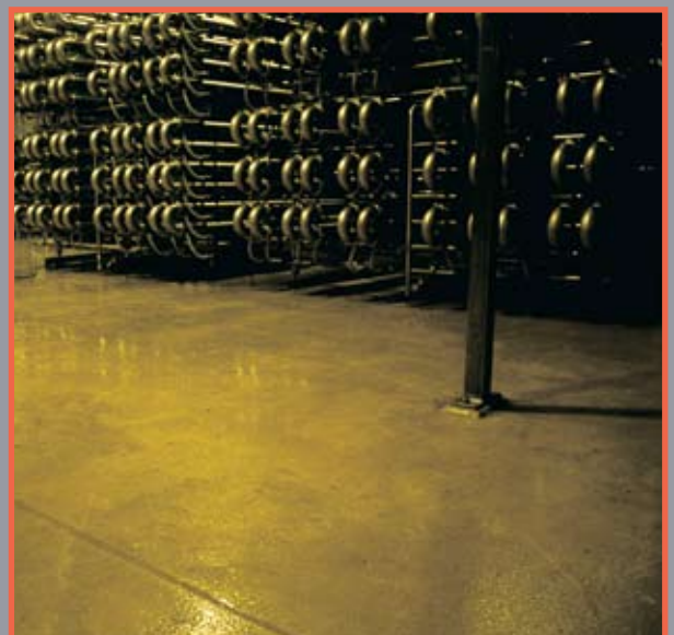
SURESHIELD FLOOR TOPPING
